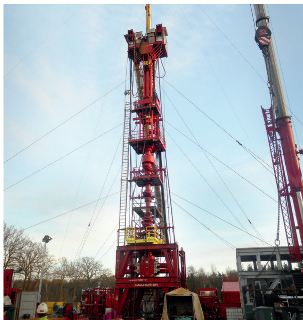
Snubbing unit used for workover services
